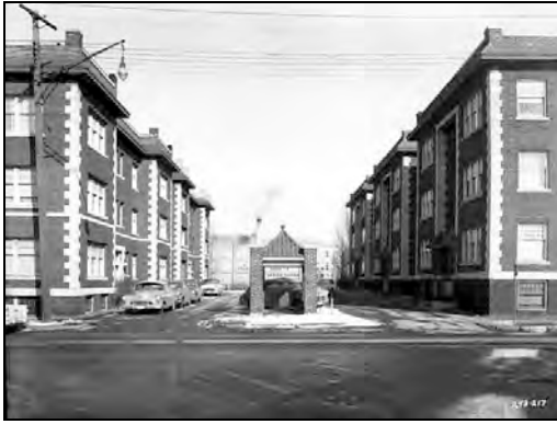
Lagoon Apartments, 2870 Holmes Ave. S. (1915) in 1957
