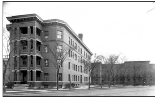
Vermont Apartments, 902 Franklin Avenue (1907, MHS). Franklin Heights Apartments (1902) are at rear.
